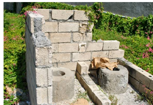
Previous latrine for 450 students+ faculty
