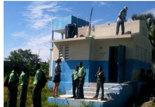
The (now) fully functioning latrine
