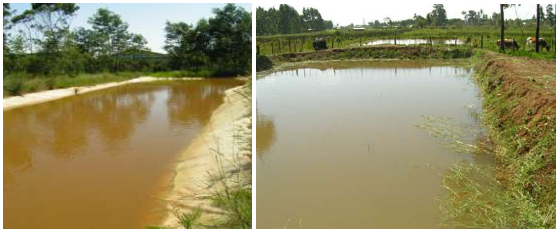
Photo 7 Pond construction near Eldoret
