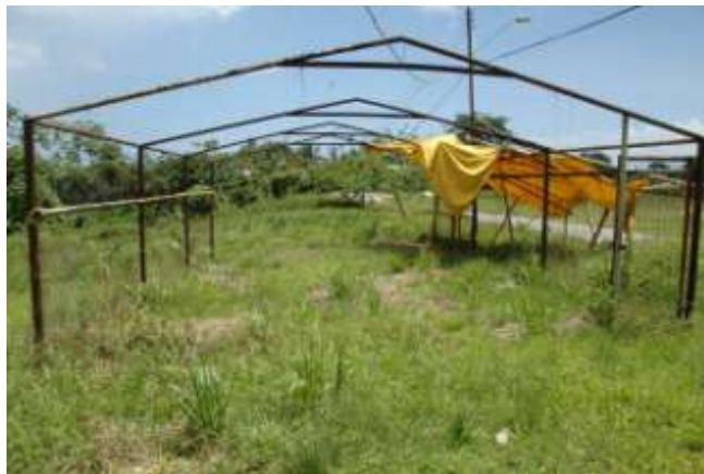
Greenhouse frame at Point Coco
