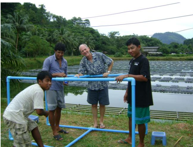
Seaweed cage construction
