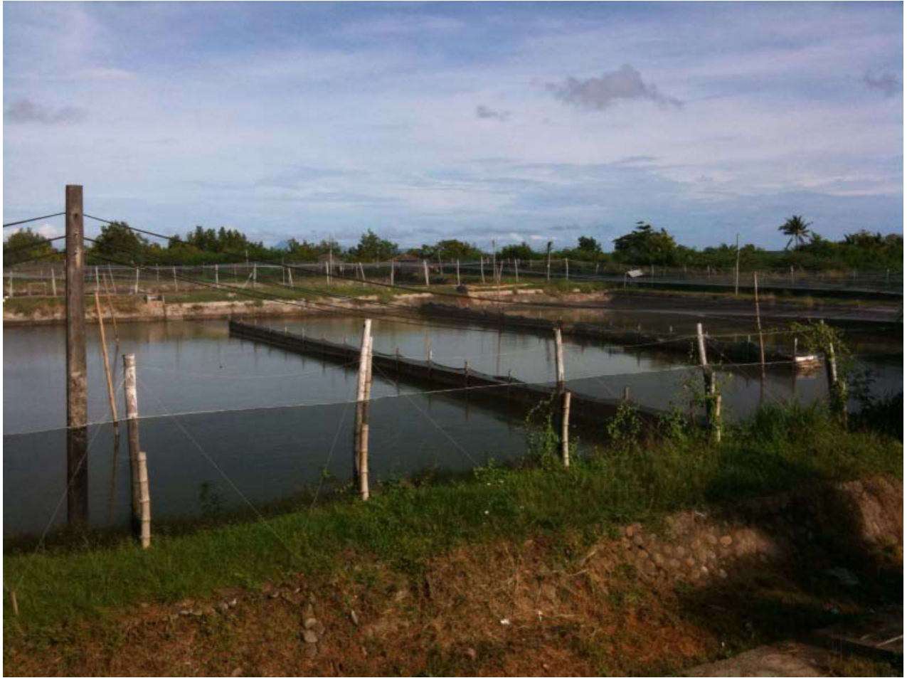
The reservoir pond for water treatment prior to flow to grow-out ponds. Note the configuration of channels to maximize settling. The water is typically screened prior to entry into the reservoir pond, settled for up to seven days, then screened again before entry into the culture ponds.
