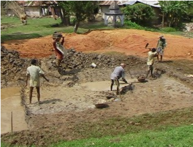
Figure 16. The dry season is the best time for digging ponds - no JCBs in small-scale aquaculture!
