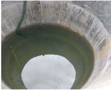
Open well for hatchery water supply
