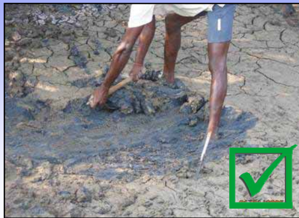
Proper removal of black soil
