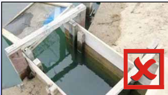
Improperly fixed water filter net
