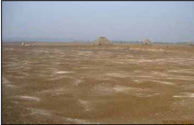
Application of lime to soil
