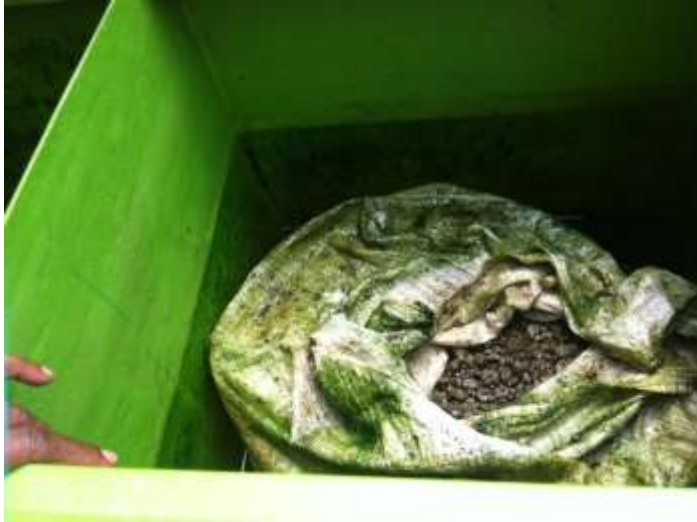
Picture 044 Sack of pumice stone currently utilized as part of the biofilter system.
