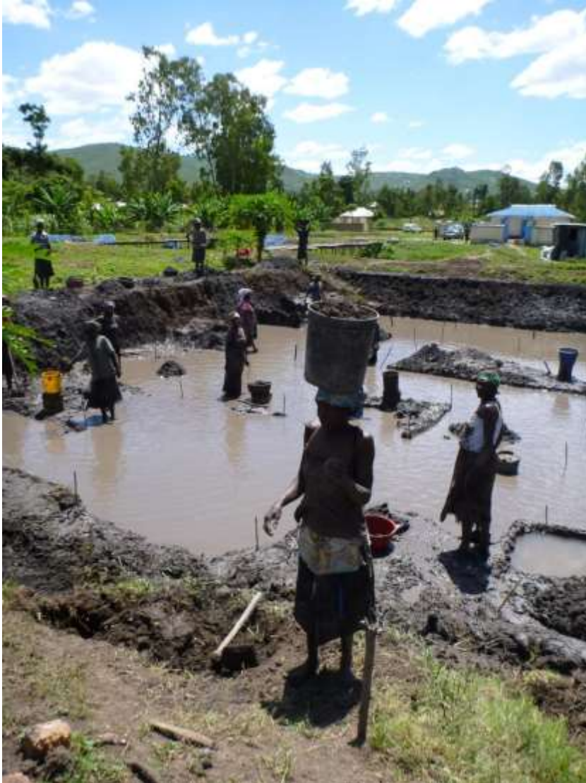
Jewlet Farm Lower Station Pond Renovation
