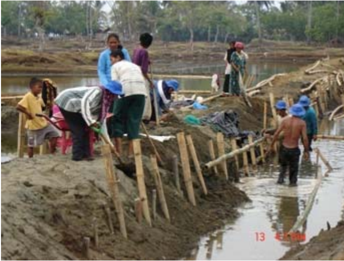
Villagers in Pasi Lhok rebuilding water supply canals damaged by the tsunami
