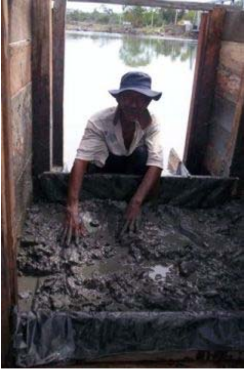
Sealing the water gate
