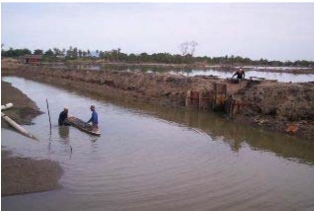
Hauling mud to seal the water gates
