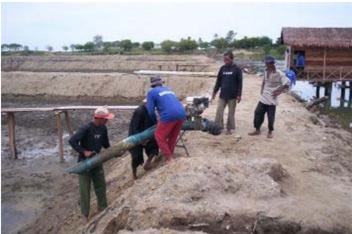
Installing the portable pump
