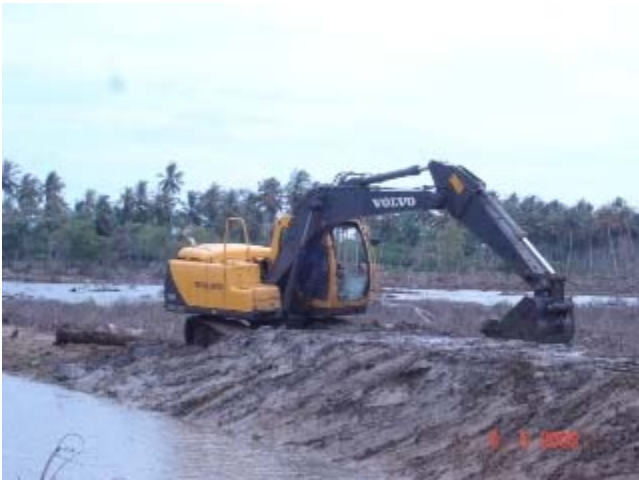
Working in wet conditions!
