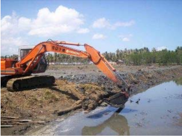
Repairing the dykes
