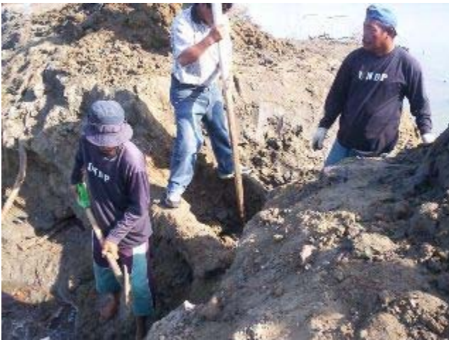
Constructing a channel for the water gate
