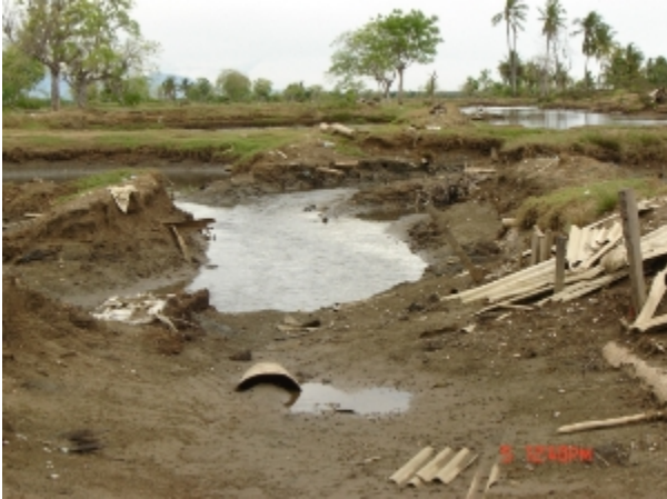
Tsunami damaged water supply canal
