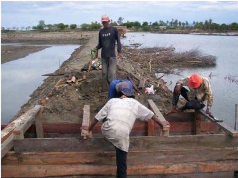
Putting the final touches to the water gate
