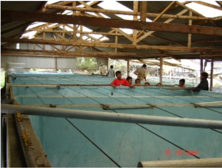
Children enjoying the new roof as it begins to take shape
