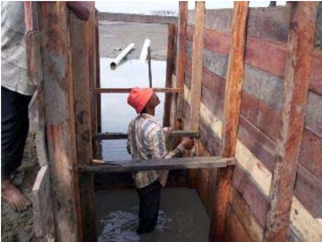
Constructing the water gate
