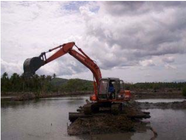
Repairing the dykes near the river
